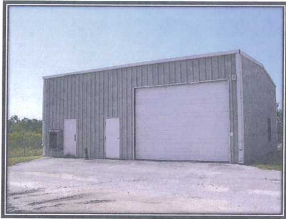
View of the metal warehouse building located along the northeastern portion of the site.
