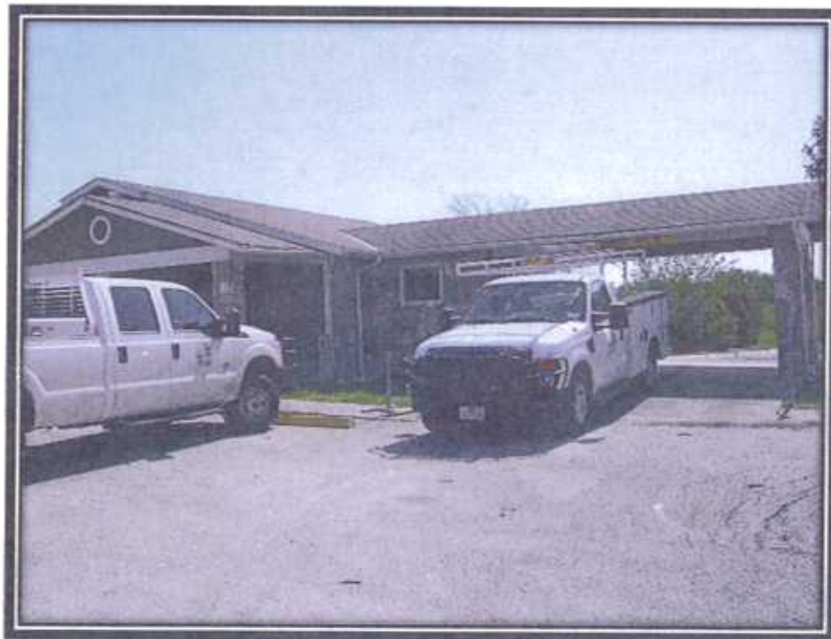
View of the drive-thru teller window located on the south side of the building.
