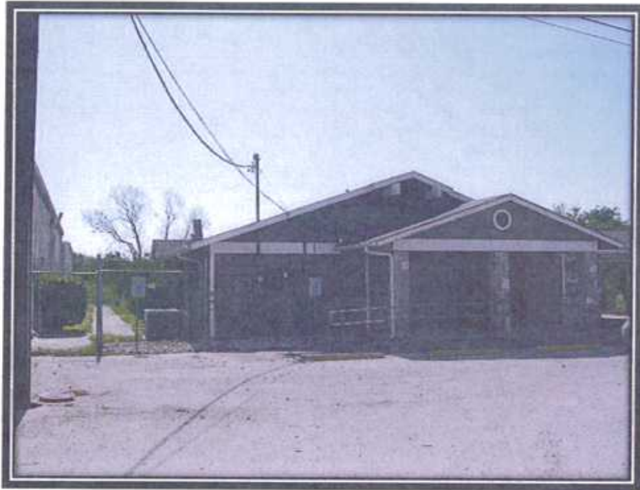
View of the front entry of the single-story office building.
