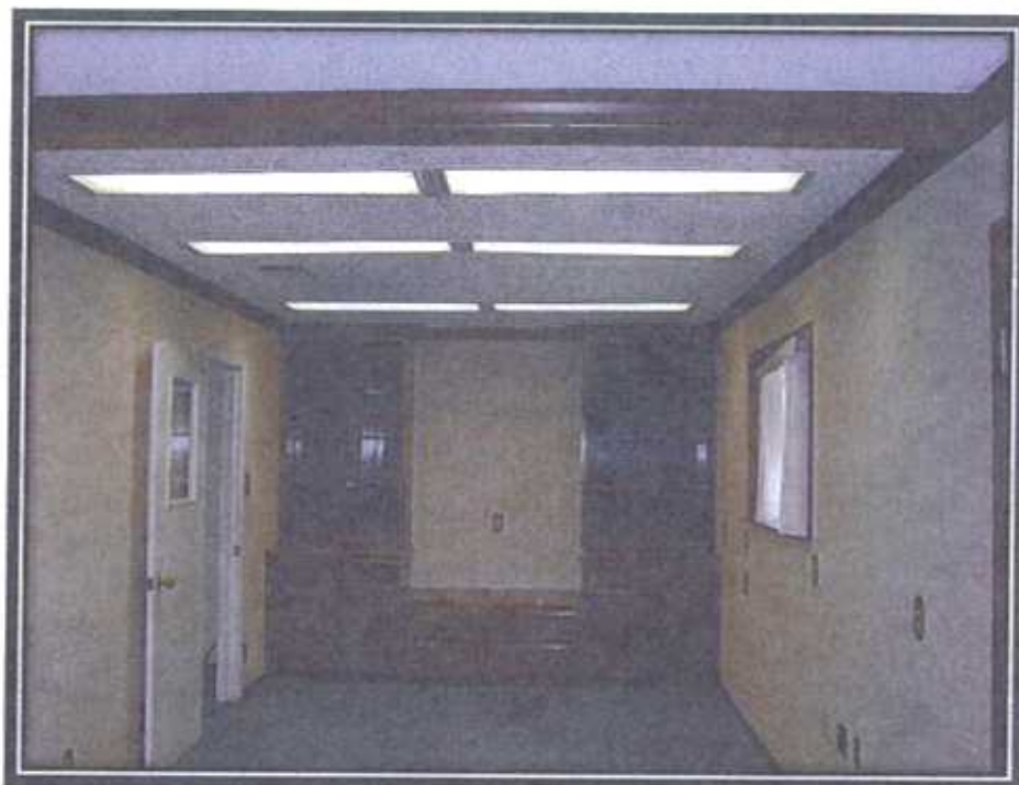
View of an office located in the one-story office building.
