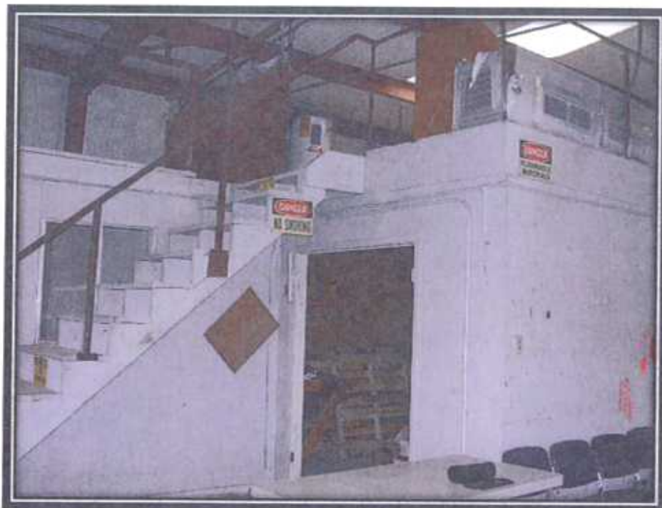
Interior view of the warehouse with stairway leading to loft area.
