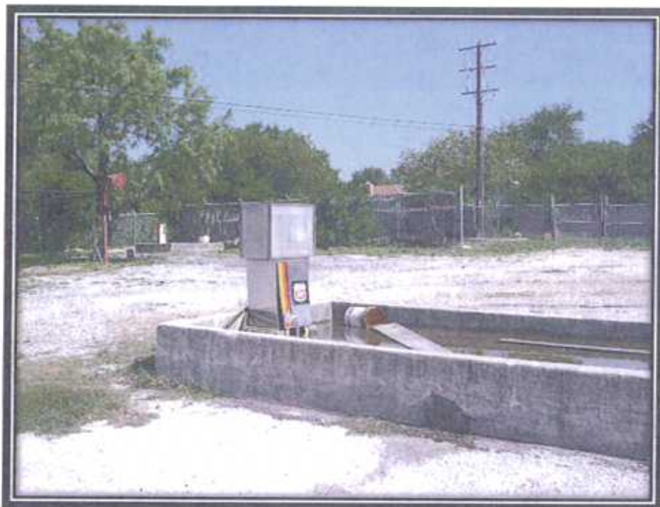
View of one of the fuel tanks looking northwest.
