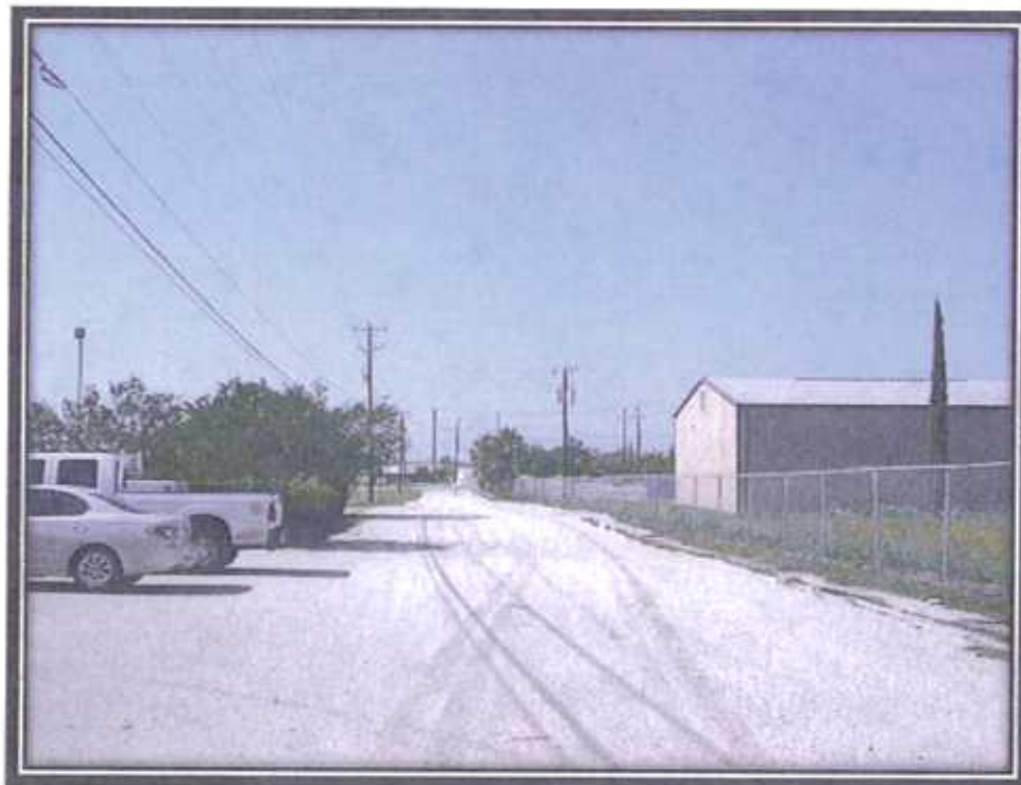
View of the driveway located along the western side of the property looking south.
